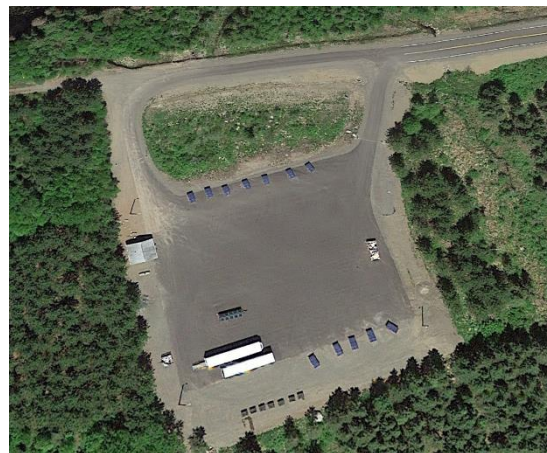
Aerial view of the Grand Portage transfer station.
