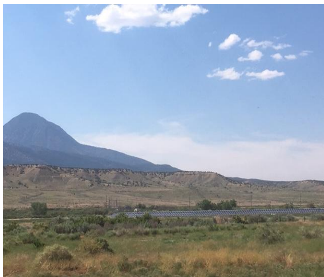
Towaoc Community Solar power plant—over 3,600 PV panels, creatively net-metered; Ute Peak in background.
