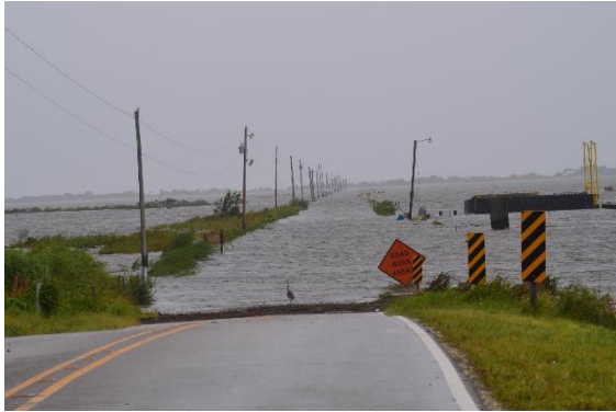
Island Road August 2020 one day after Hurricane Laura. Photo: Chantel Comardelle
