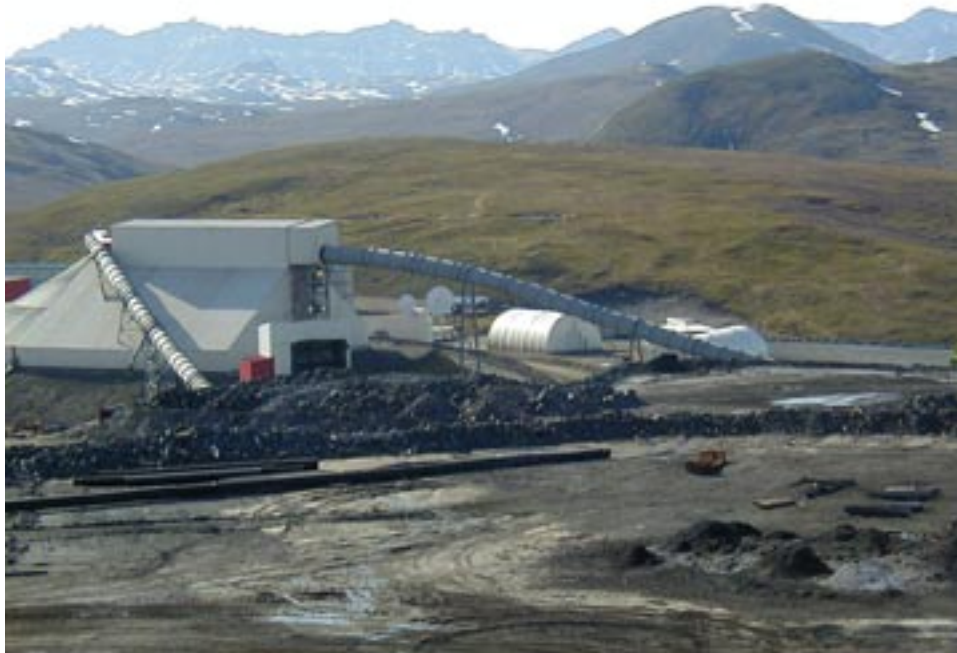
The Red Dog Mine mill where ore is processed into zinc and lead concentrate.
